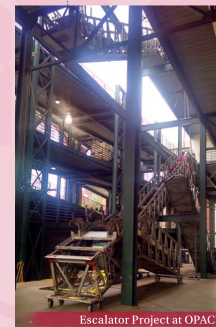
Escalator Project at OPACY
