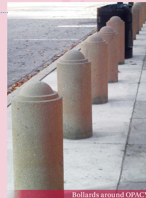
Bollards around OPACY
