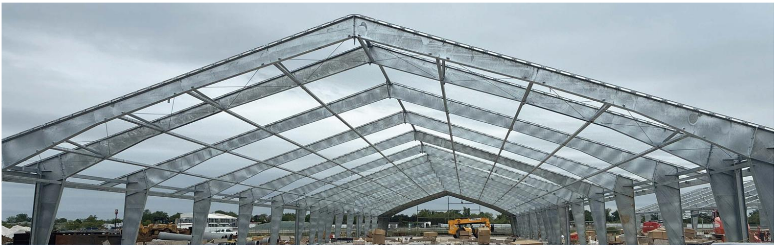
Form and framework: The new steel structure for the receiving barn takes shape at the Pimlico Redevelopment project
