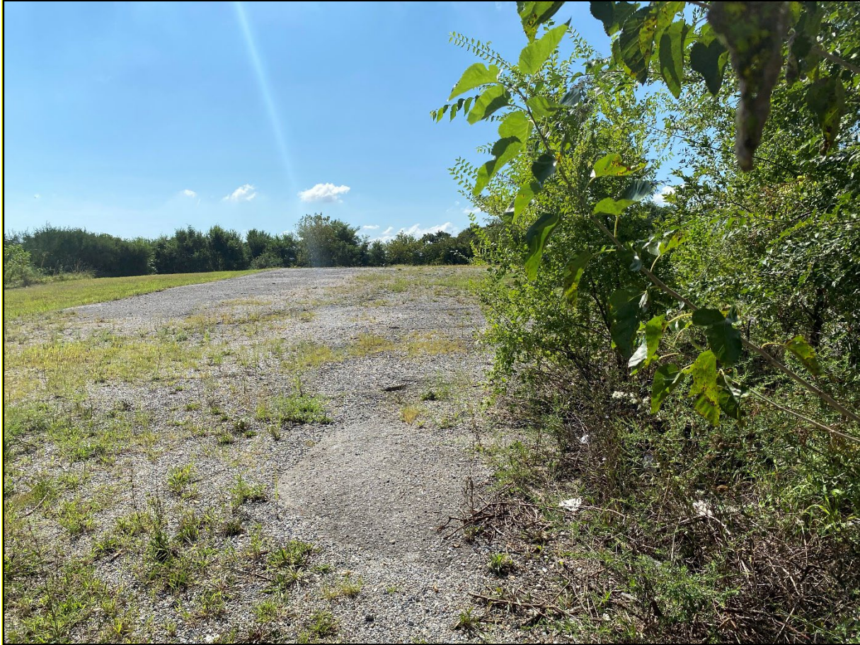
Figure 3-29. Abandoned parking lot in the northern portion of Project Site # 2, showing the gently rolling topography occupied by the pavement. View to the east.
