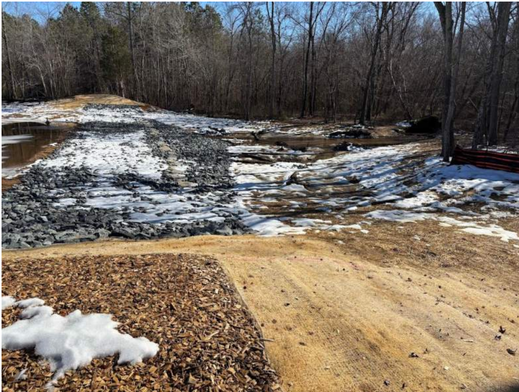
Photograph 1: View of gravel access road, facing east
