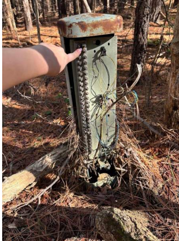
Photograph 5: View of Utility Box, closed, facing southeast
