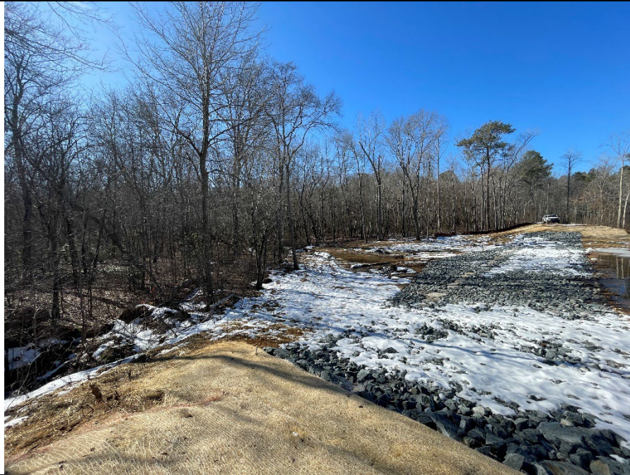
Photograph Number 9: Facing southwest St. Mary's River within the center extent of the PSA.
