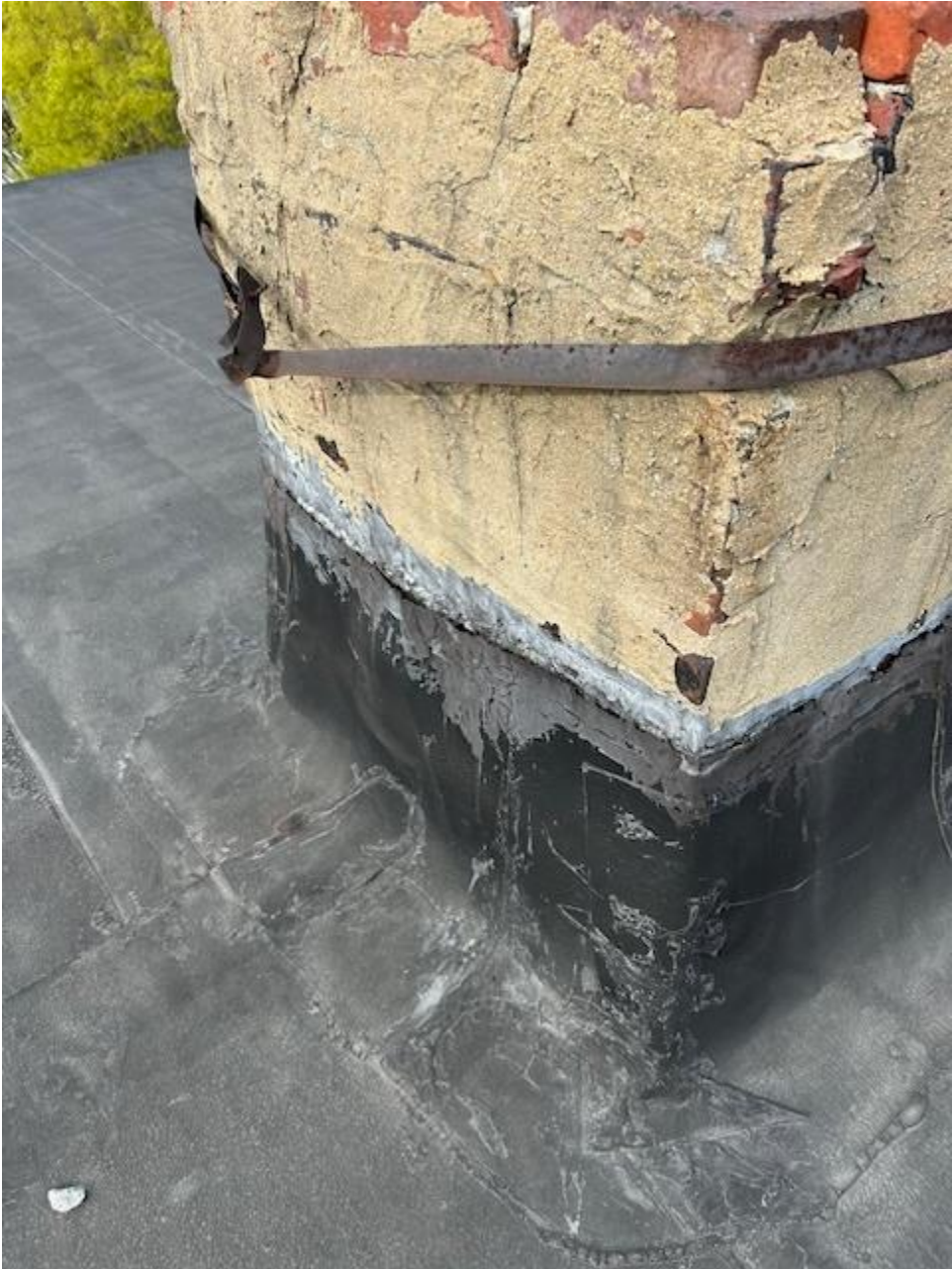
Chimney flashing
