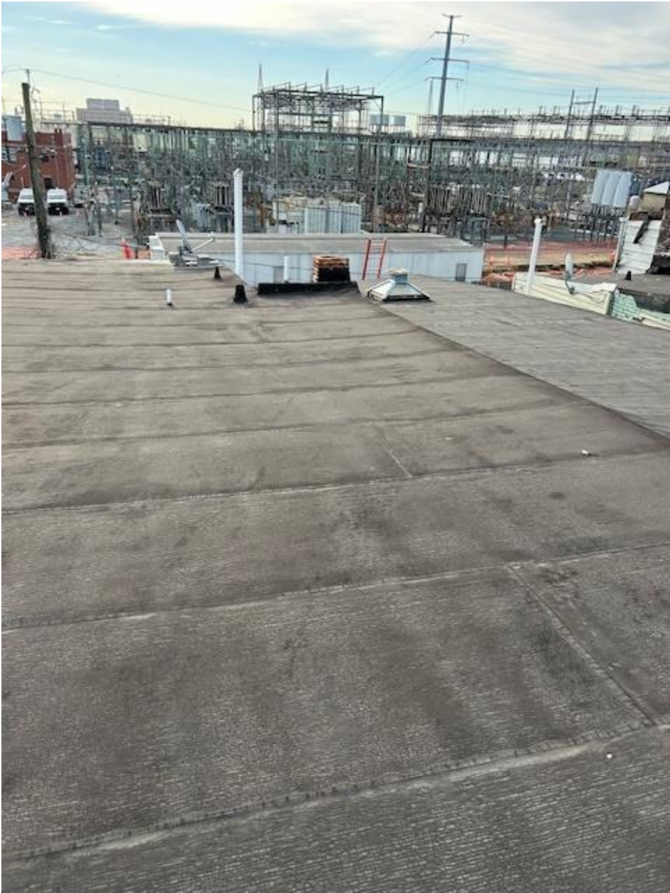
2009-2013 Annapolis Rd, Rooftop
