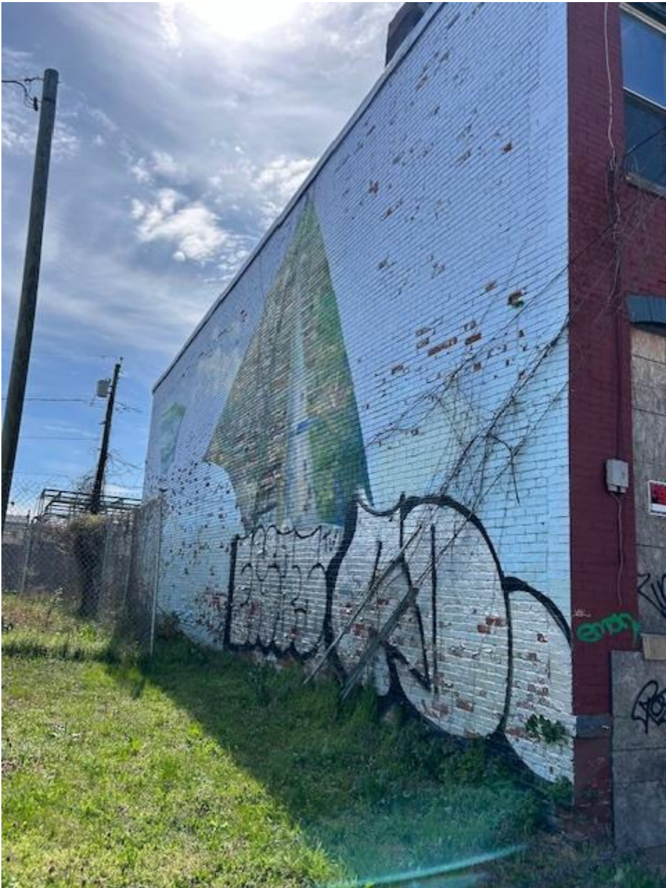
2009 Annapolis Rd. Side wall
