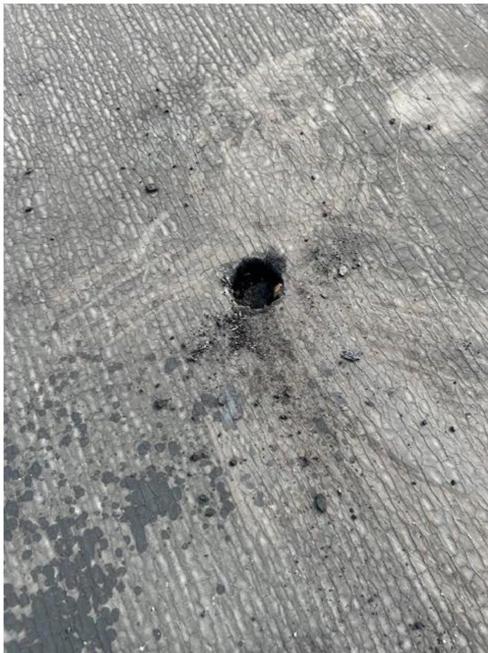
Roof sample location
