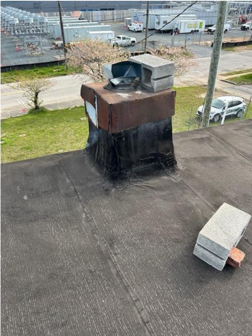
Chimney flashing
