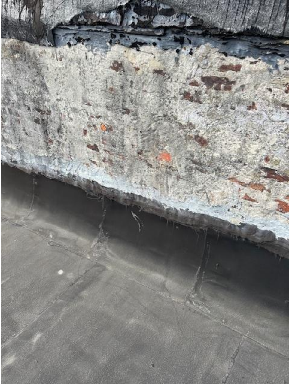
Roof and wall flashing
