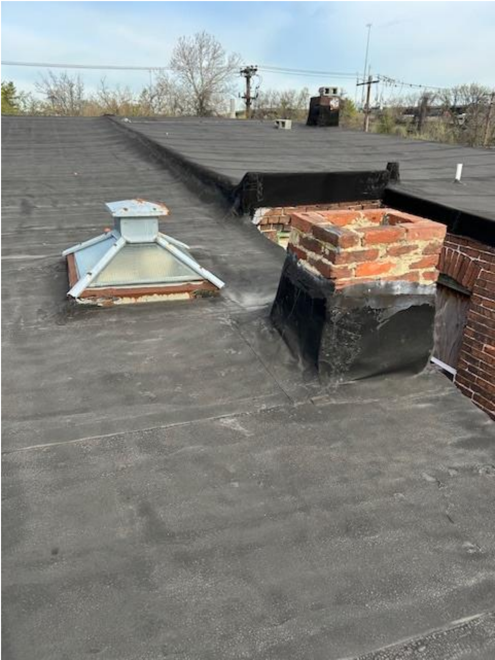
Chimney flashing and Skylight
