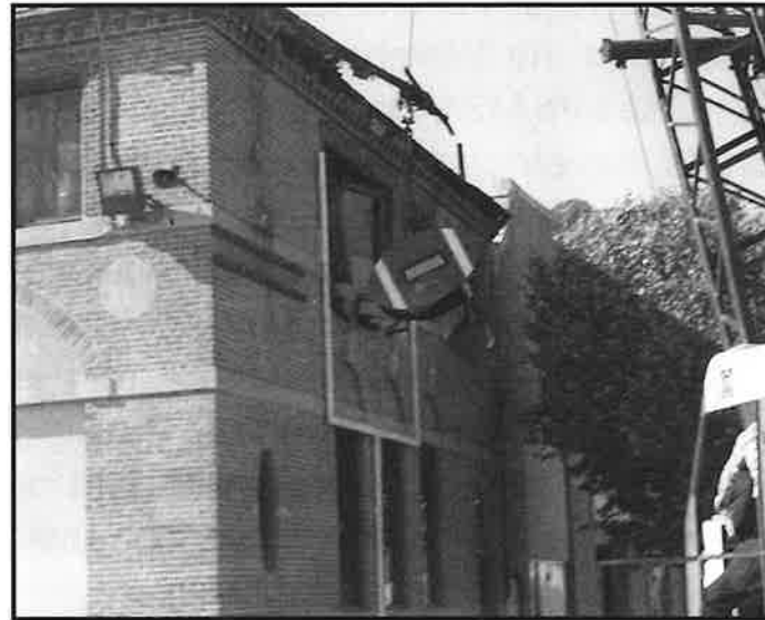
The wrecking ball begins demolition of Hammerjacks
