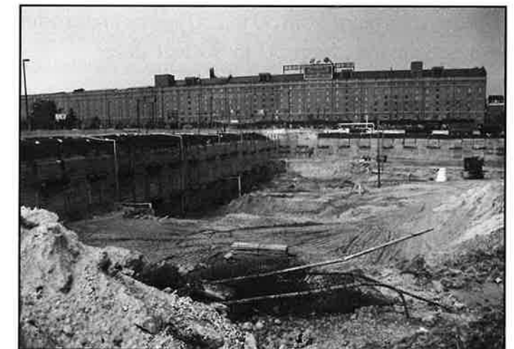
EXCAVATION OF BALTIMORE CONVENTION CENTER EXPANSION (LOOKING WEST)
