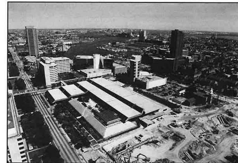
AERIAL VIEW OF BALTIMORE CONVENTION CENTER EXPANSION PROJECT
