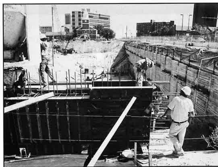
WORKERS ERECT HOWARD STREET FOUNDATION WALLS
