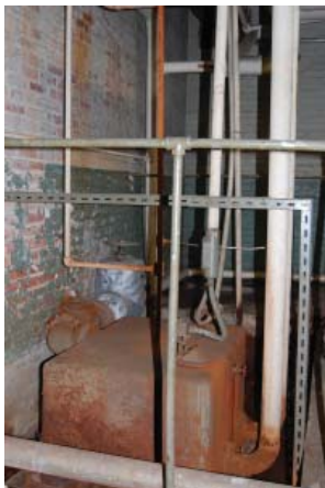
Corroded Water Pump in Courthouse East
