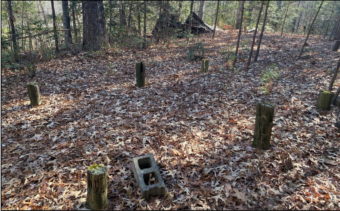
Figure 3-15. Wooden piers and nearby structure demolition debris associated with former structure location north of the identified cellar hole, view to the southeast.
