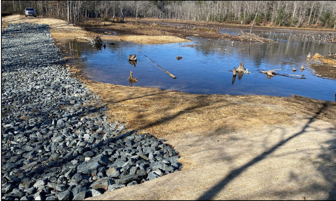
Figure 3-16. Overview of recently constructed spillway on southern edge of Johnsons Pond, view to the northwest.
