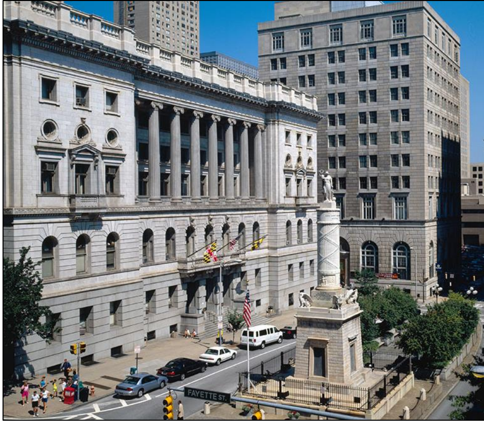
Front Elevation Facing East to Calvert Street
