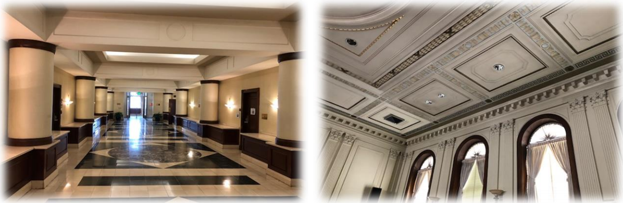
Typical Interior Views of Courthouse East
