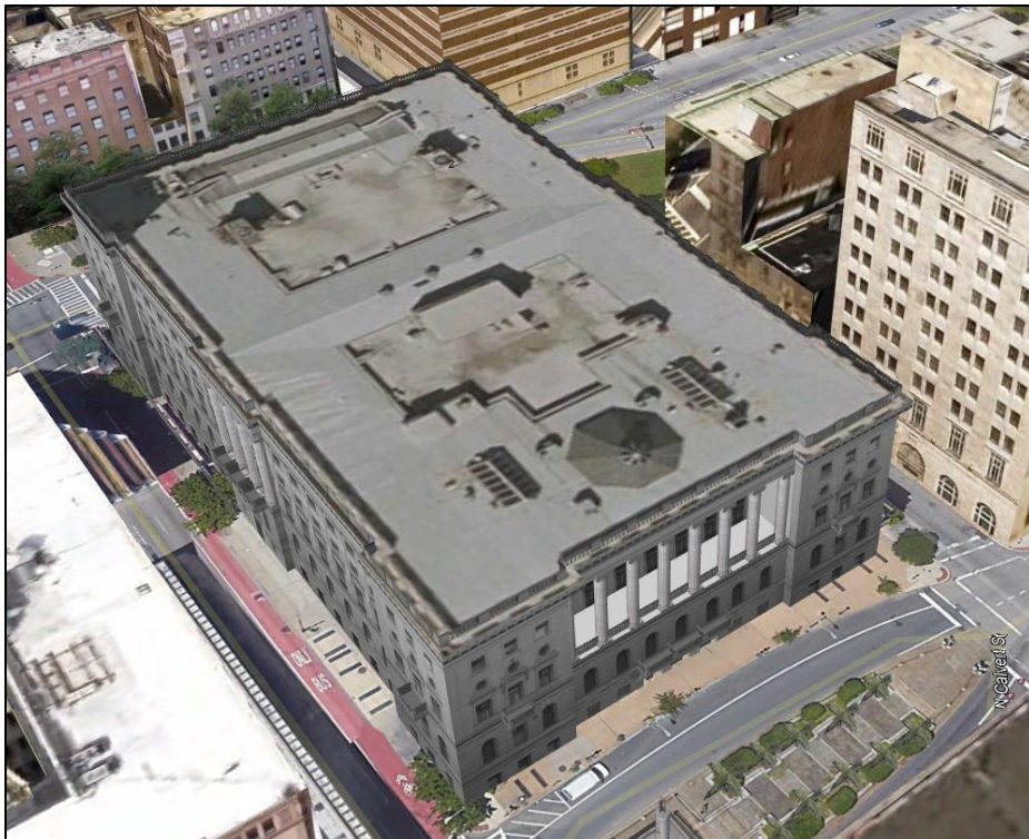
Aerial View Looking Northwesterly at Front Elevation
