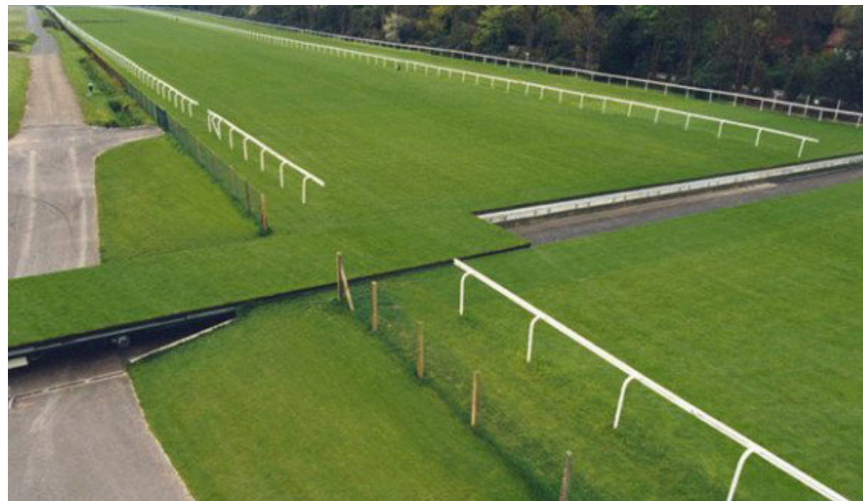
Ascot turf track road crossing utilizing tray system
