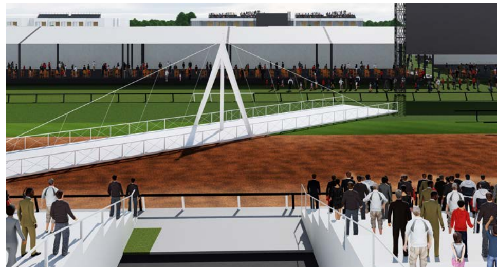
Center pivot pedestrian bridge - opening in progress
