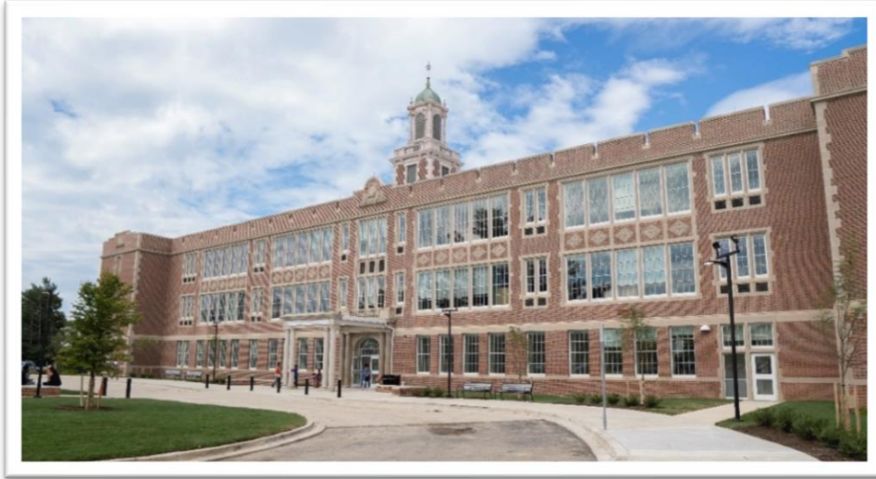
Figure 5. Robert Poole Building Exterior
