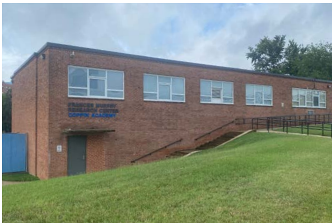
Grade change adjacent to Coppin Academy
