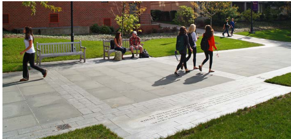
Example of scored concrete in ashlar pattern with bluestone or concrete unit paver banding. The University of Scranton Royal Way Inscription.
