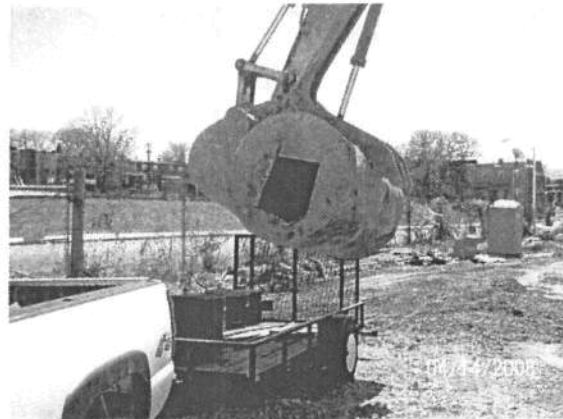
Photograph 12: Loading Heating Oil Tank for Disposal
