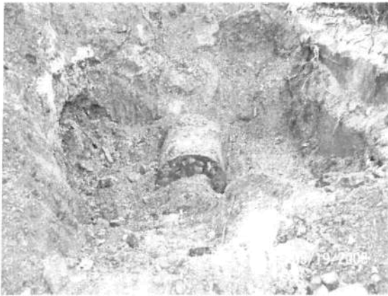
Photograph 3: Heating Oil Tank Prior to Removal
