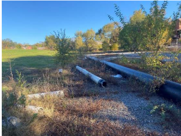
Figure 8. Pipes remaining on site November 3, 2022.
