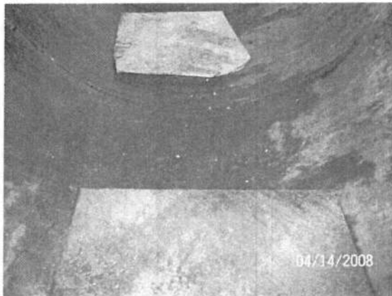
Photograph 11: Heating Oil Tank Cleaned
