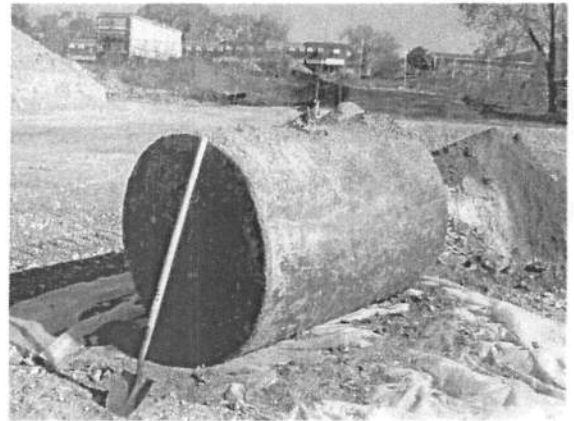
Photograph 6: Heating Oil Tank Removed Prior to Cleaning
