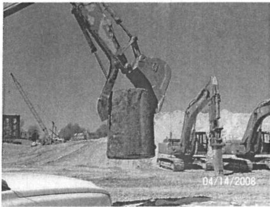
Photograph 13: Loading Gasoline Tank for Disposal
