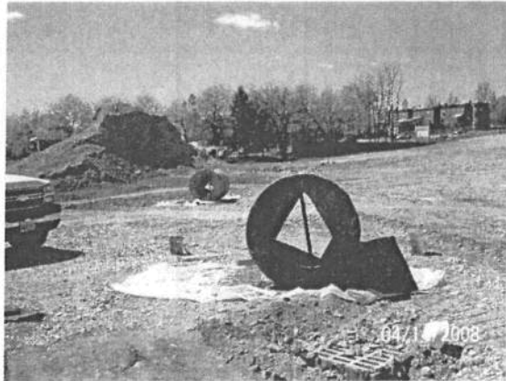
Photograph 9: Both Tanks Cut and Ready for Cleaning
