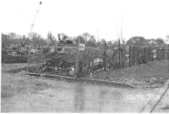
Photograph 1: Entrance to work area
