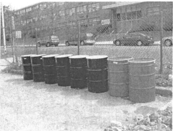
Photograph 15: Drums Containing Water and Sludge from Oil and Gasoline Tanks Ready for Shipment
