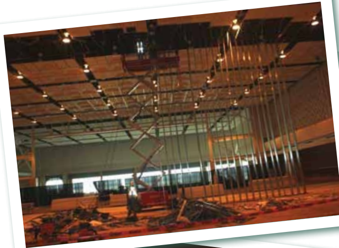
Work begins on the new Performing Arts Center.
